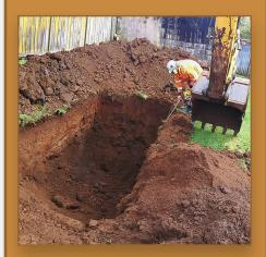
Test pits are dug to determine the geology and the water table of that site, are usually between 3 and 12 feet deep, and are dug either by hand or by using a mechanical digger. Some of the reasons for a test pit are standard penetration test, permeability tests, pile integrity tests (see February's newsletter), and sample series tests.
